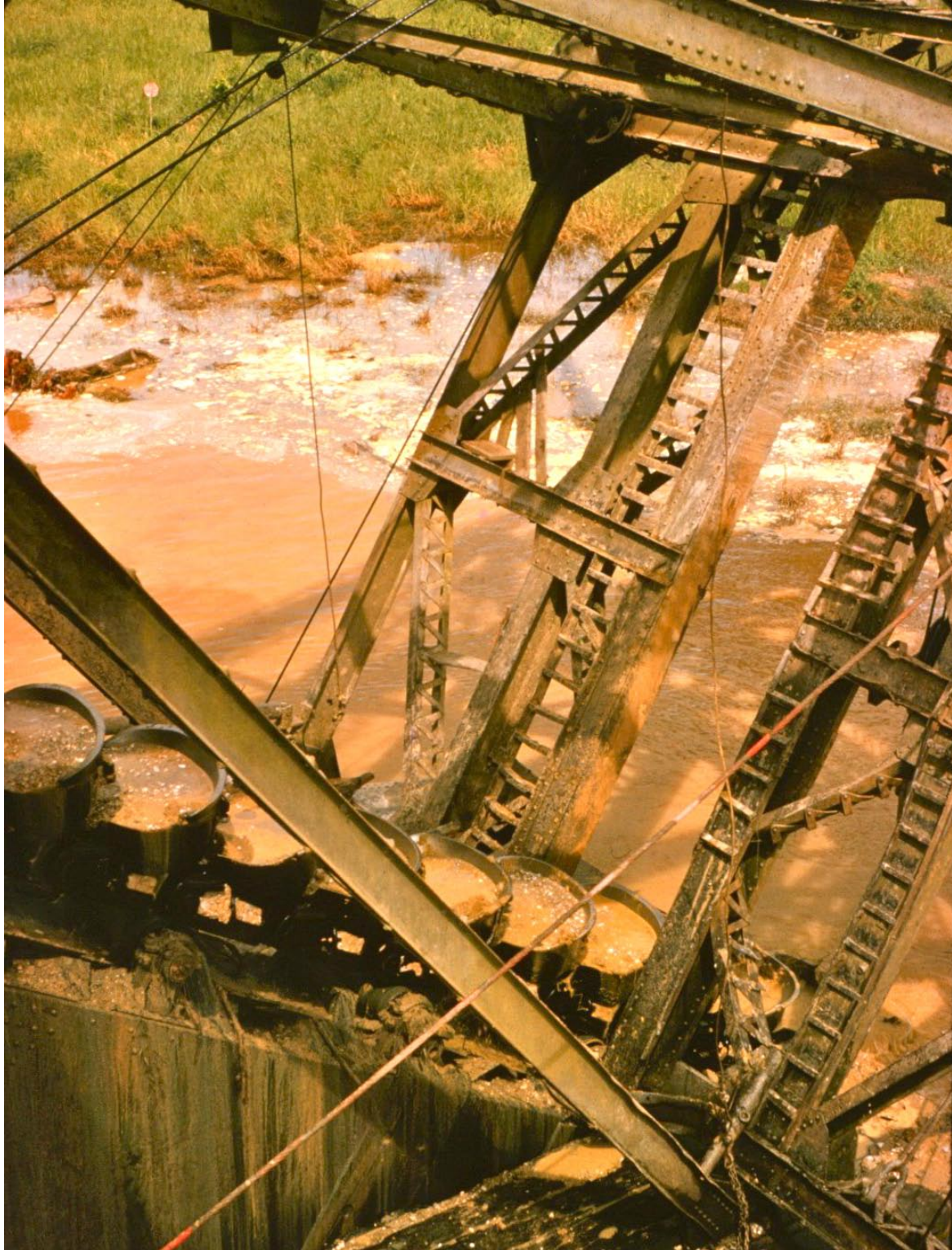
Figure 6. Gravels excavated from Offin River Valley are lifted onto Bremang Gold Dredge using large steel scoops attached to a conveyor, during 1963 operations
